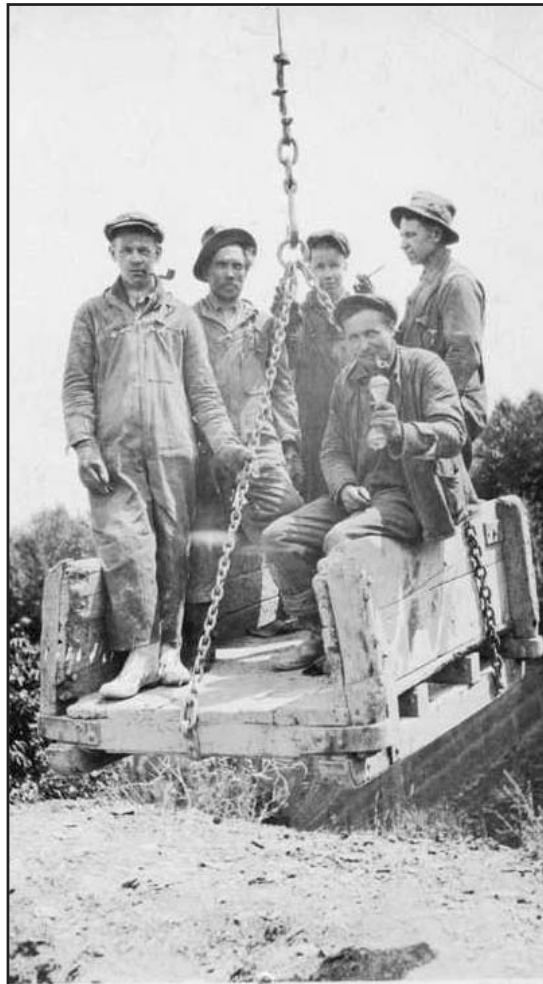
Five Monson-Maine Slate Company quarry workers in a wooden hoist box ready to be lowered into the quarry to work, ca. 1910. Contributed to the Maine Memory Network by the Monson Historical Society.
